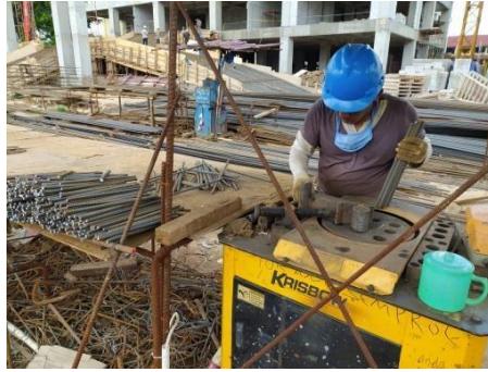
Gambar 2.17 Bar Bending
